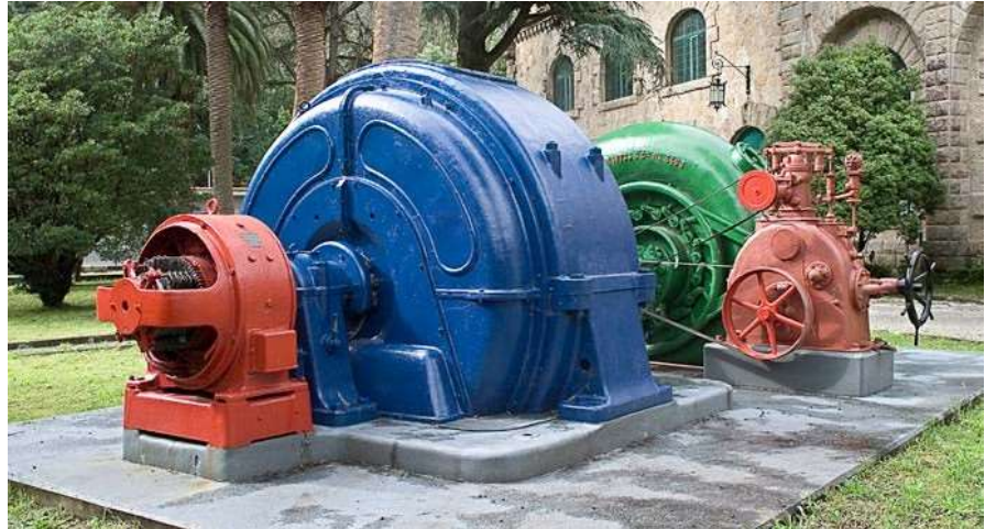
Image 12: Dynamo of the old Tambre I power station, exhibited for museum purposes in front of the main façade of the power station.
