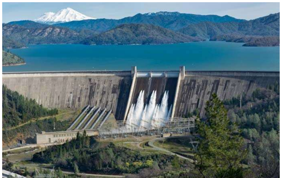
Image 92: Photograph of a reservoir.
