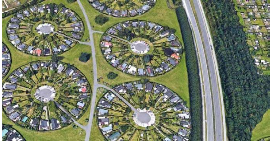
Image 112: Brøndby Haveby (Denmark).
