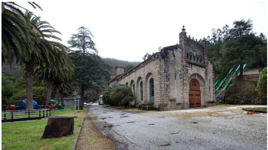
Image 11: Tambre I Power Station - Noia (A Coruña). Built in 1932 and designed by the architect Antonio Palacios using Galician historicist architecture applied through a Romanesque-style façade transferred to an industrial building.
